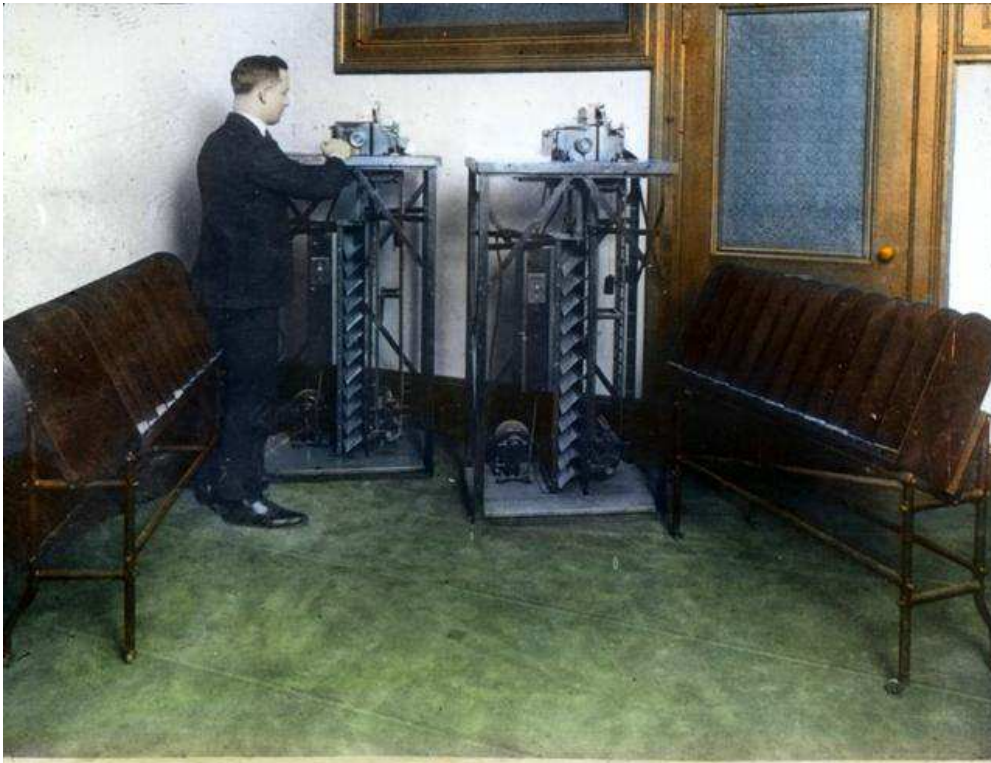
One operator and two Electric Sorting Machines can distribute cards into predetermined classifications at the rate of 500 every minute
